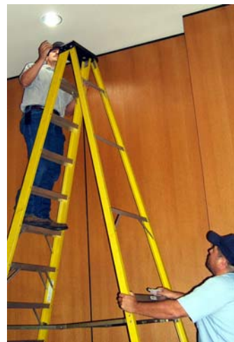
On October 4 Facility Services staff replaced 52-watt bulbs with 20-watt fluorescents that produce 75 watts. Rene Fuentes (left) and Johnny Hernandez (right) made the change in council chambers.
